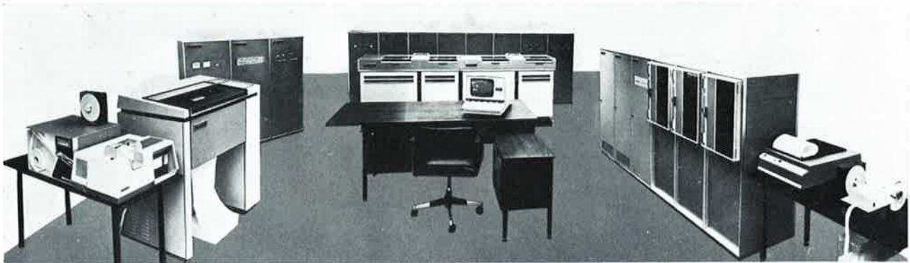
Figure 4: Panorama of the NORDIC installation.
